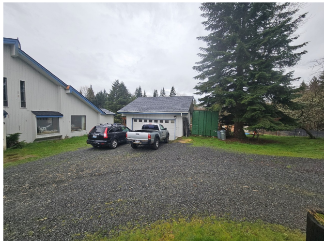
Photos 11 & 12 (Map Photo ID 301): Main residence and garage, looking south. A creosote retaining wall was located just behind Photo 12.
