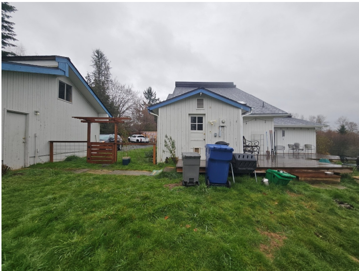
Photo 14 (Map Photo ID 289): Western side of the main residence, looking east.
