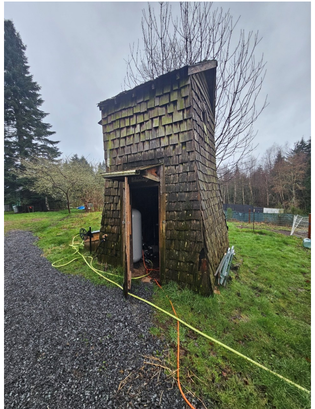
Photo 8 (Map Photo ID 284): Well house, covering well equipment and a dug well.
