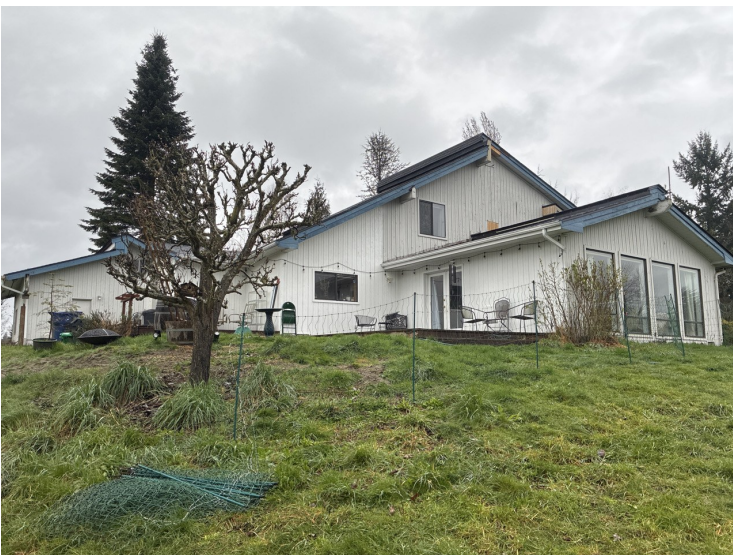
Photo 15 (Map Photo ID 291): Southern side of the main residence. From here, the property slopes south to the Stillaguamish River. Septic field is just downhill and right (east) of this photo. Septic access is buried.
