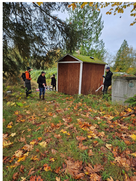
Photo 11 (Map Photo ID 179): Current construction of the new well pump house. The previously used concrete cistern can be seen on the right. The new well is located directly south on the neighboring parcel, across 246th St NE.
