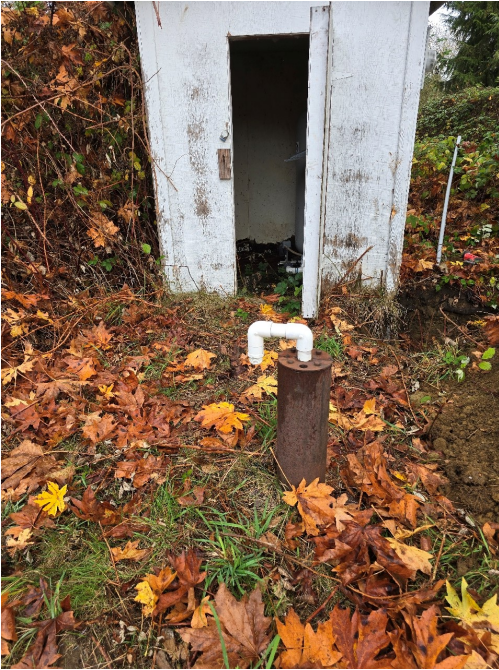
Photo 12 (Map Photo ID 180): Old well house and well, just west of the new well/pump house.
