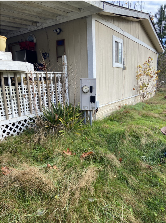
Photo 1 (Map Photo ID 208): The electric meter located on the Southwest corner of the primary residence.
