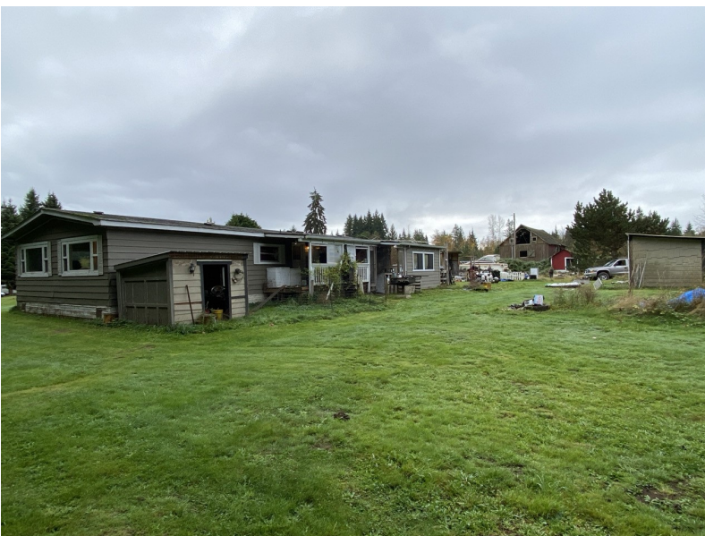
Photo 21 (Map Photo ID 157): Looking at the western side of the house, towards the large piles of junk along the southern property line.
