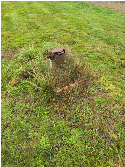
Photo 3 (Map Photo ID 148): Drilled well on the parcel, near the driveway along the southern property line.
