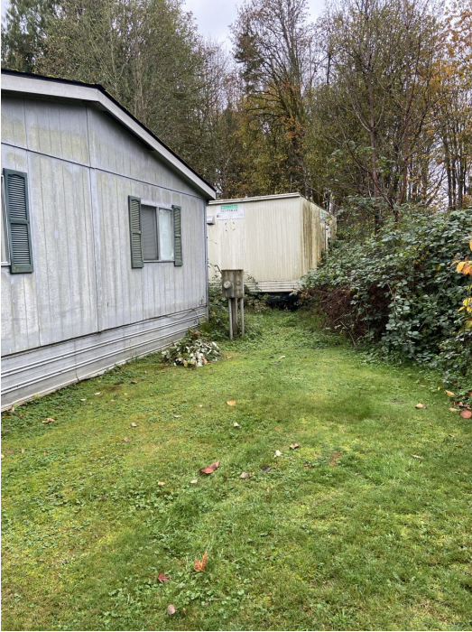
Photo 3 (Map Photo ID 236): Electric meter, north side of the house, and a trailer in the background.
