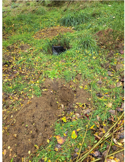
Photo 14 (Map Photo ID 140): Dig and fill areas near the center of the southern property line.
