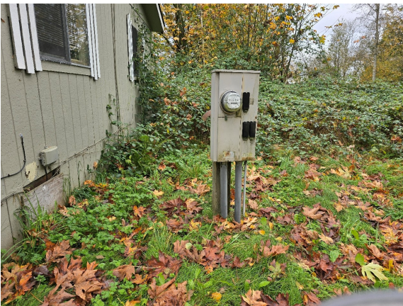
Photo 4 (Map Photo ID 223): Electric meter on the north side of the house.
