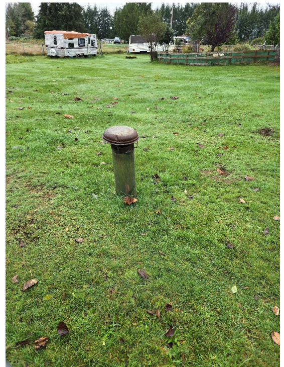
Photo 7 (Map Photo ID 118): Old chimney pipe that appears to be stuck in the ground. This was inside the fenced backyard and staff were unable to investigate further. Two old trailers can be seen, as well.
