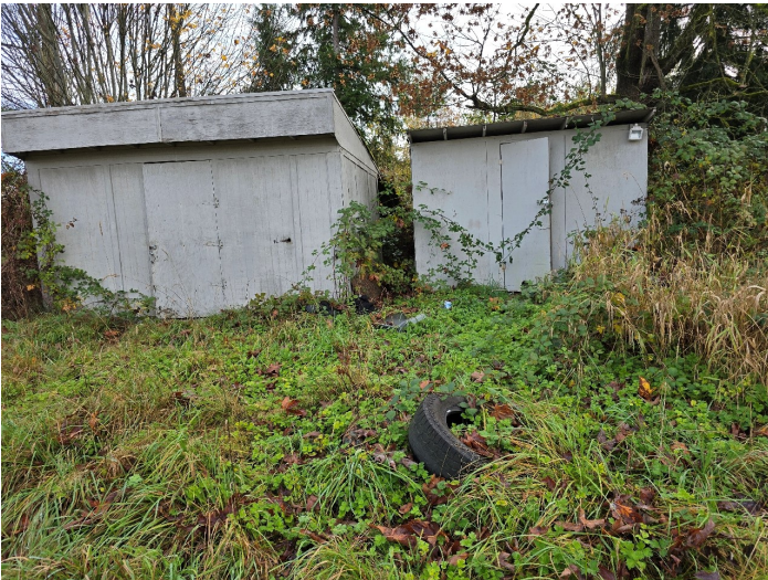
Photos 4 (Map Photo ID 215 ): Just south of the house, two storage sheds filled with junk and old chemicals.
