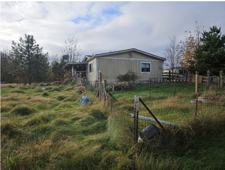
Photo 4 (Map Photo ID 203): The northeast corner of the house, looking southwest.
