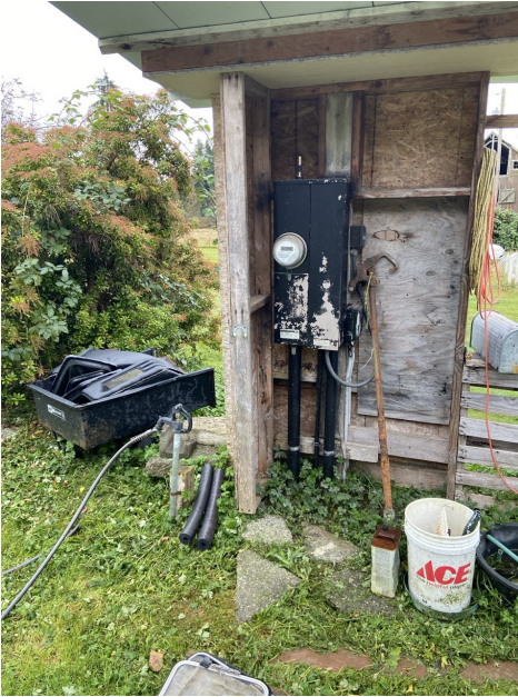
Photo 15 (Map Photo ID 168): Electric panel protected by a partial enclosure located on the southern side of the house, near the center of the property.
