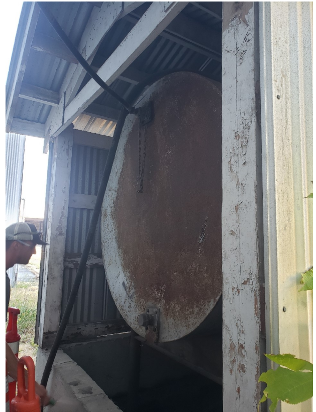
Photo 11: The backside of the [right] shed featured in Photo (6). A large, empty fuel/oil tank was found. This tank sat on top of a concrete 'tub', sealed on all sides, including the bottom. There was a small amount of hydrocarbon contaminated soils inside the concrete tub. Map Photo ID: 49.
