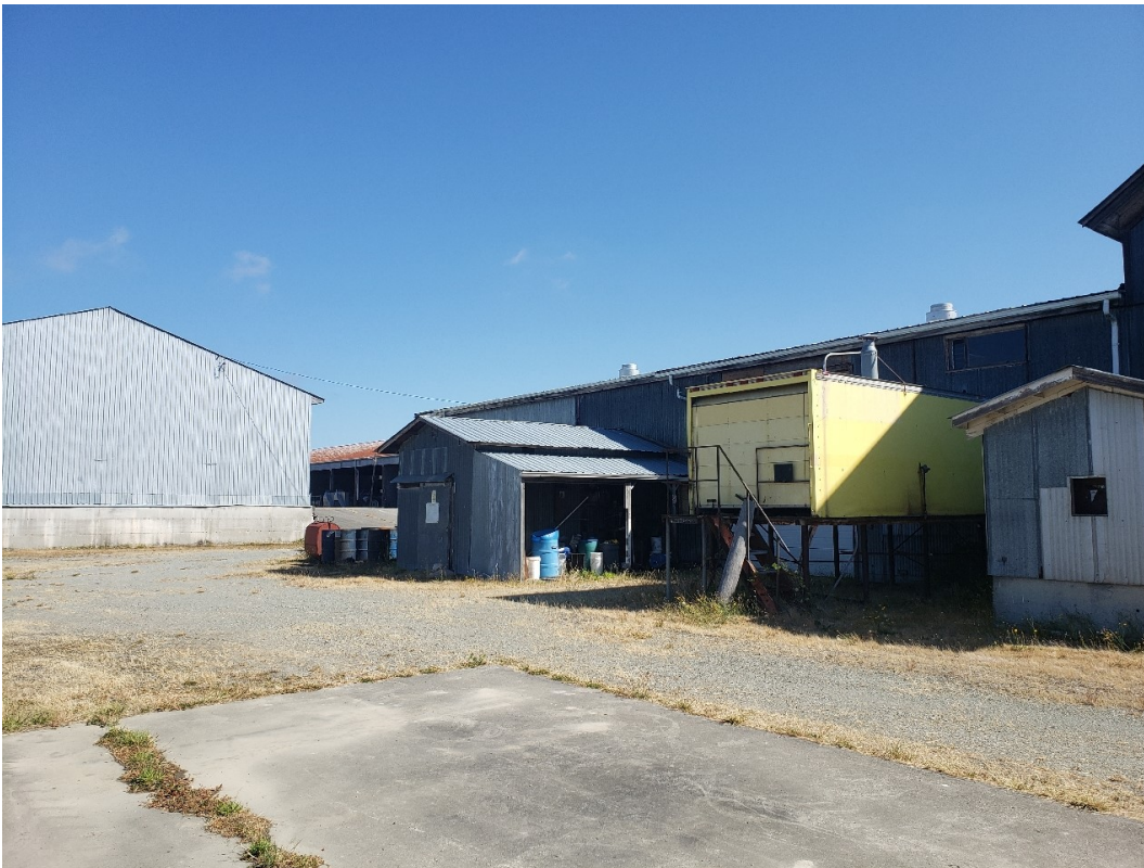
Photo 6: The western side of the north shop. The door to enter the motor oil storage room seen in Photo (5) can be seen to the right of the 55-gallon drums. This photo depicts a storage area of used 55-gallon drums, an oil filter recycler (open-air shed on the left), a semi-permanent building which houses a large air compressor (yellow structure), and another fueling station (shed on the right). Map Photo ID: 56.
