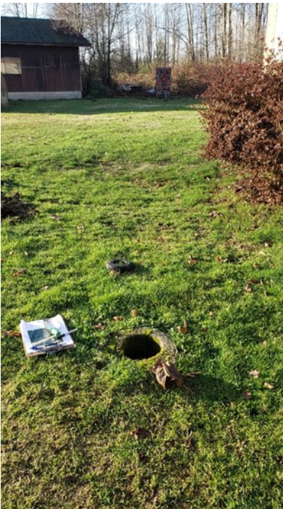
Photo 44: On the south side of the mobile, a concrete hole/pipe was located. Likely irrigation infrastructure, but nothing was found on the inside.
