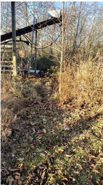
Photo 19: Filled in sawdust loading ramp previously discussed in Photo (13).
