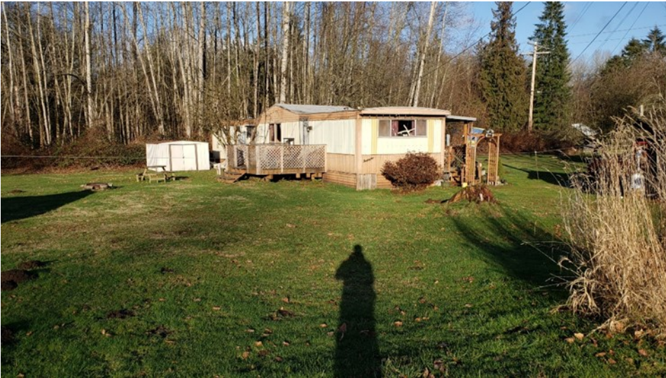
Photo 43: The backside of the mobile, looking north.
