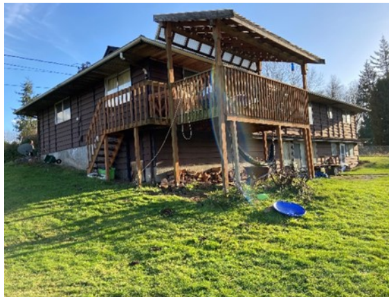
Photo 2: The main residence from the backyard. The water treatment infrastructure is located under the stairs—water filter, conditioner, etc. can be found in this room. Photo taken looking south-east, towards 15 th Ave.
