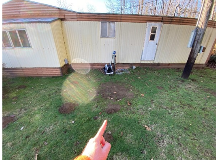
Photo 47: Approximate location of the septic tank for the mobile, located on the eastern side of the building.
