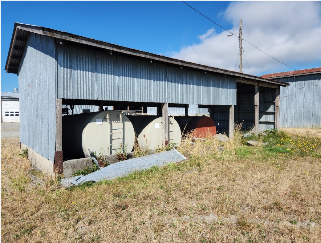
Photo 19: A large fueling shed for farm activities. At the time of survey all three tanks were empty. They historically contained red dye diesel (farm diesel), unleaded petroleum, and hydraulic fluid. The two bays not occupied were believed to have been used for other fuels and/or fluids. The tanks were inside a concrete tub and no apparent oil contamination was visible around the shed. This fueling shed is just to the south of the historic barn. Photo was taken looking northwest. Map Phone ID: 32
