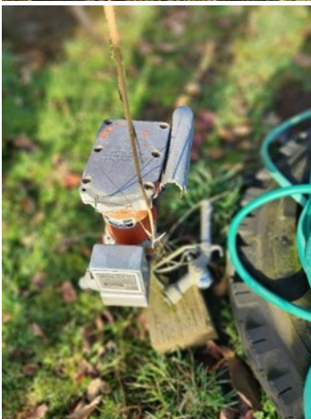
Photos 23 & 24: Next to the garage, there is an Underground Storage Tank containing gasoline. Owner claims the tank was likely pumped out by his father following the closure of the mill. However, the vent pipe smelled like product was still present. The tank is presumed to be 4-5' long and 3' wide.
