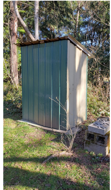
Photo 8: A homebuilt smoker located just to the northeast of the chicken coop. Photo taken looking northeast
