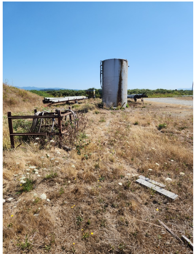
Photo 28: An old water tower and pipes found just north of the pole barns. A small hill can be seen to the left, likely created by dug material from ditching efforts that occurred across the property. TCF vegetable processing water was piped from the main facility, under the river, around this hill, to the two irrigation ponds in the southern portion of the property. Photo taken looking east. Map Photo ID: 81
