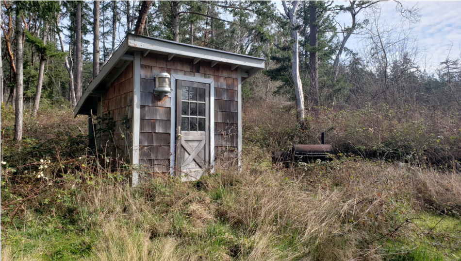
Photo 7: A small outbuilding, behind (north) the residence. This outbuilding houses a washer/dryer and hot water tank. Additionally, a small charcoal grill was found just to the east of the outbuilding. Photo taken looking northeast
