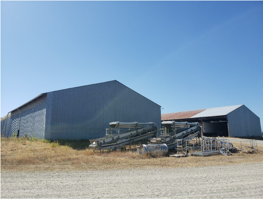
Photo 29: The north side of the two pole barns. TCF was using this location to store surplus equipment, no HAZMAT was located in this area. Photo taken looking south. Map Photo ID: 84.1
