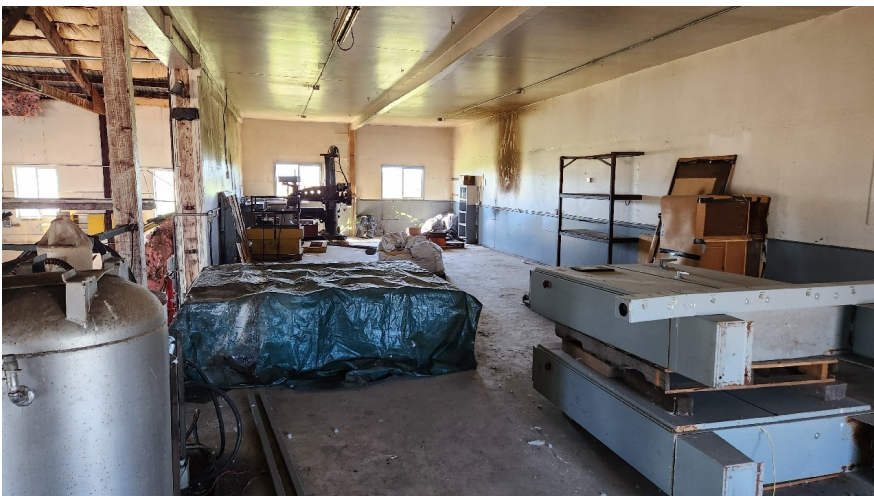
Photos 32-34: The eastern portion of the second shop. This area of the shop had loose and falling insulation, extensive bird and rodent feces, and oil stains on the concrete floor. It hadn't been used in years. Various large equipment, cabinetry, chemicals, were located, along with a second industrial sink (draining location unknown). Map Photo IDs: 68.2, 68.3, and N/A (sink).
