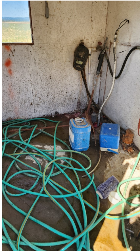
Photos 14 and 15: An outbuilding that was used for an unknown purpose. Currently, it stores a welding mask, grease gun, hose, and some containers.
