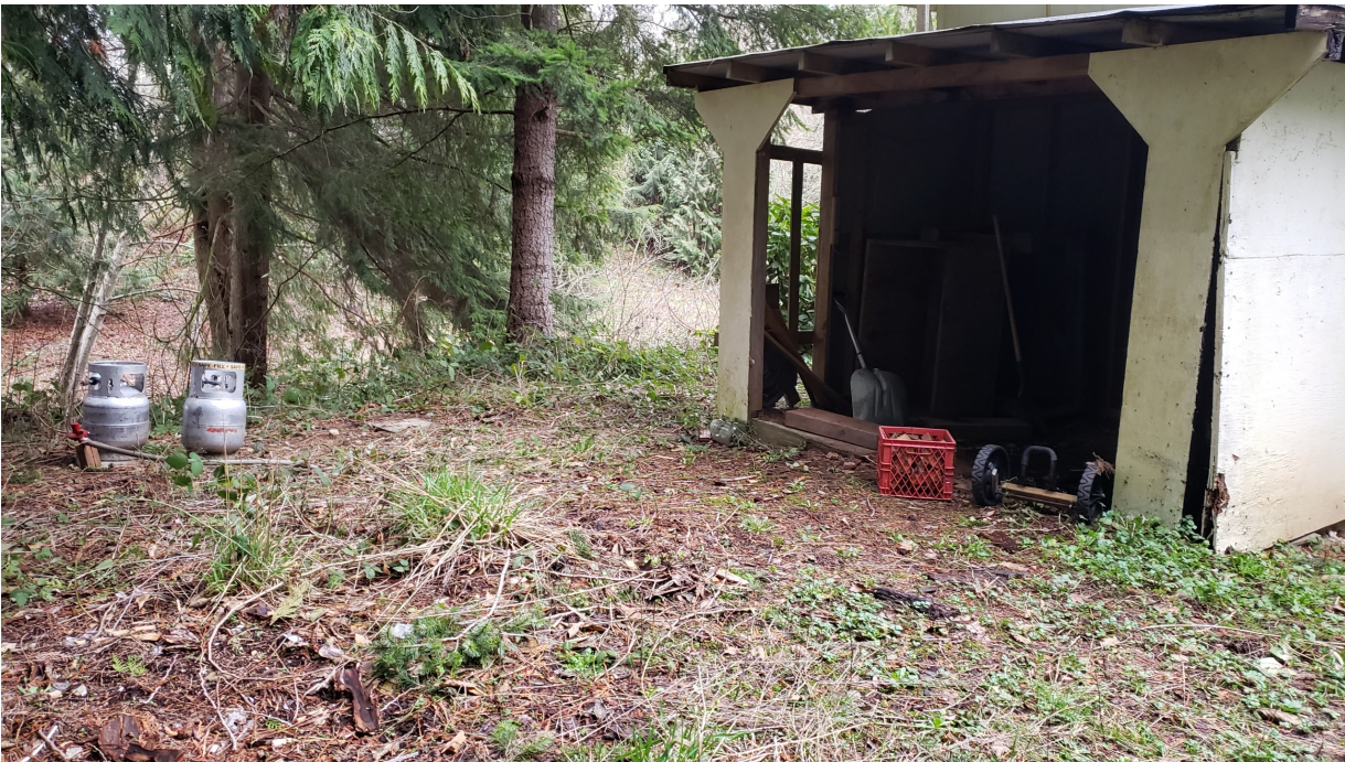
Photos 33: A shed attached to the western side of the main residence. Additionally, two propane tanks can be seen. The owner installed pipe to provide propane into the main residence.
