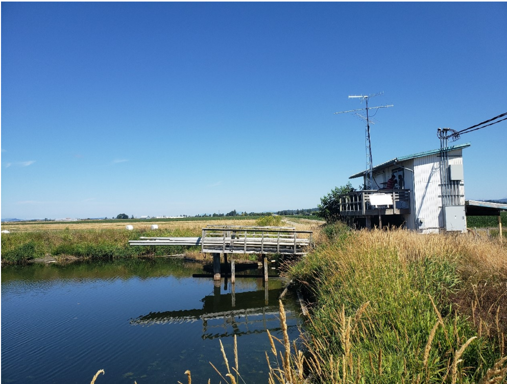
Photo 40: The pump house located at the southern and oldest irrigation pond. Vegetable processing water from TCF would be pumped into these ponds, then pumped out to fertilize/irrigate the fields. This is also the location of a Stillaguamish Tribe MOTUS tower. These ponds were built on the lowest elevation portion of the property (historic tidal wetland channel). The large barn off Thomle Road pictured in Photo (39) can be seen in the distance. The pump house is approximately 1 mile from the main, developed portion of the property. Photo taken looking north. Map Photo ID: 95.1
