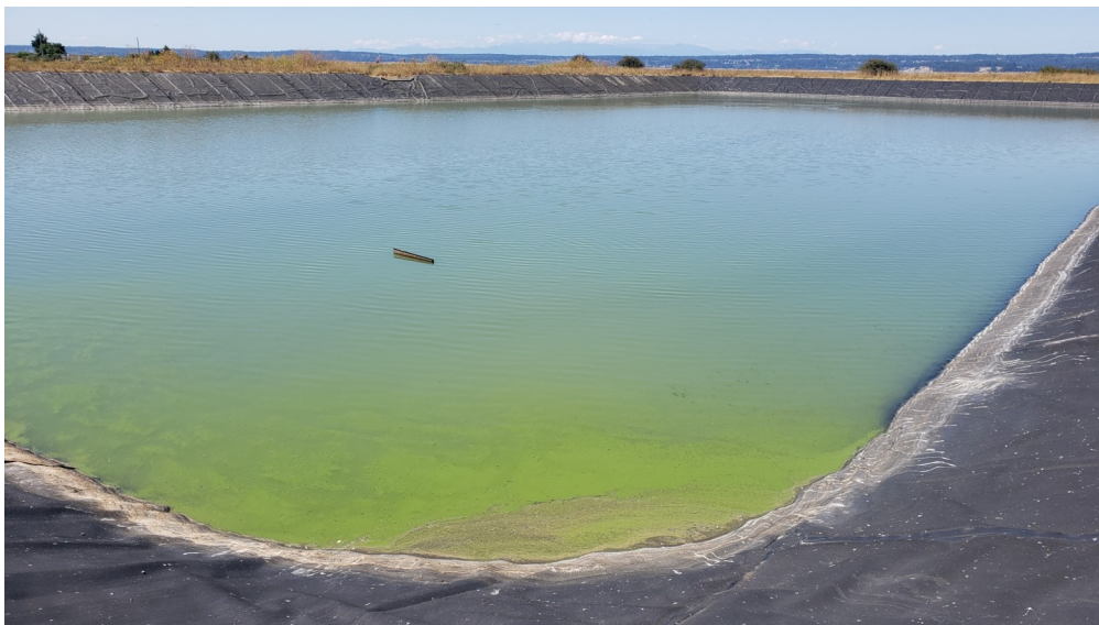
Photo 43: The second, newer and lined irrigation pond, just south of the other pond. This pond is approximately 100 yards long. Steve Karcher believes an underground pipe can fill this pond from the other, likely passively as both ponds are near the same elevation. Staff were unable to verify the presence of an underground pipe. Photo was taken looking south. Map Photo ID: N/A
