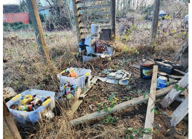
Photos 16 & 17: Various buckets and containers of grease, oils, and other chemicals underneath the mill.
