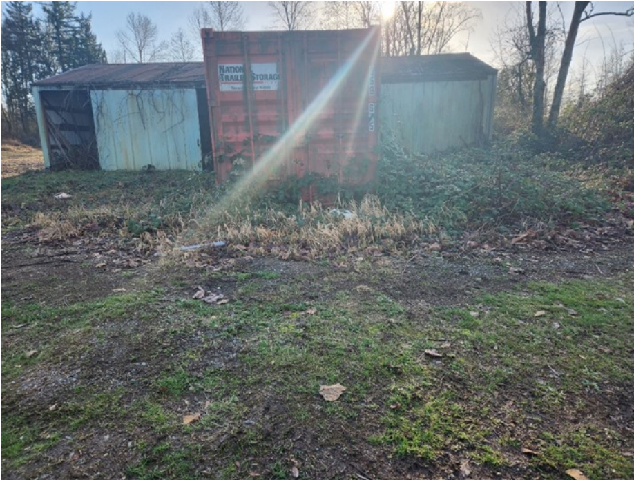
Photo 39: Shingle/shake finishing building, along with a conex storage container.
